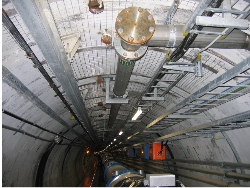
Figure 6.54: View of sector 4 showing the chain of superconducting magnets in the arc.
